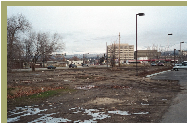
Brownfield sites can be prime redevelopment properties.
