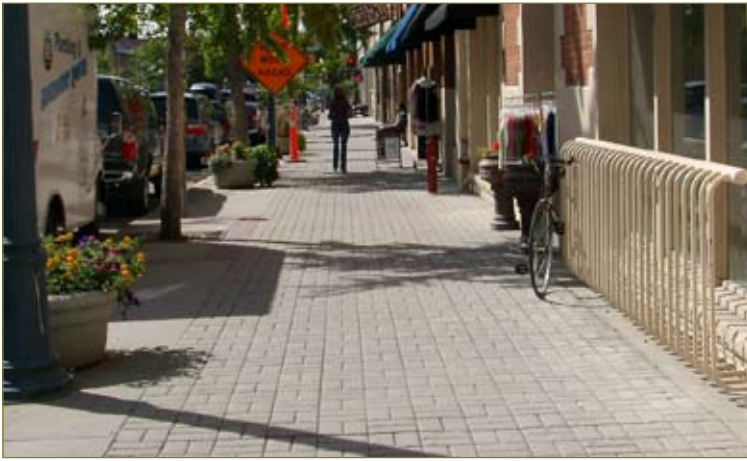
One of the main needs in the area is to replace the stamped concrete sidewalks that present an accessibility barrier and don't conform to downtown design standards.
