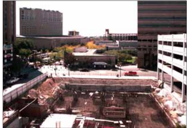
Boise Tower site at 8th & Main streets.
