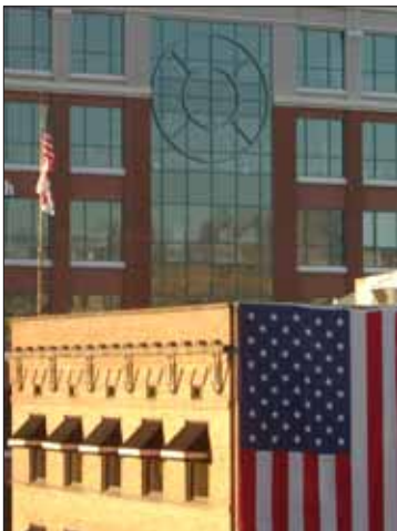
The McCarty Building shines in front of the 9th & Idaho Center
