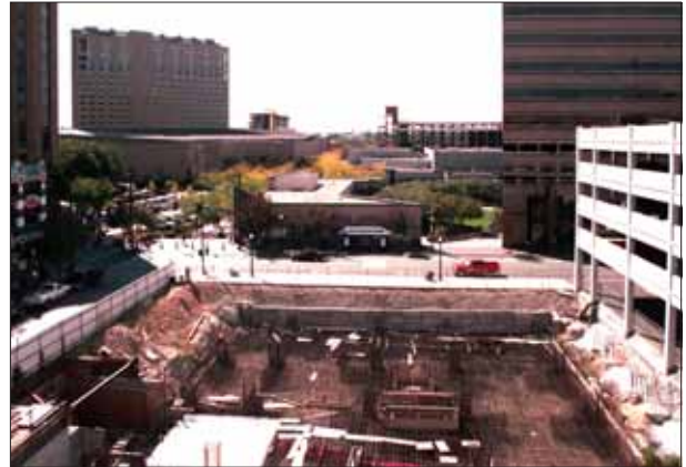
Boise Tower site at 8th & Main streets.
