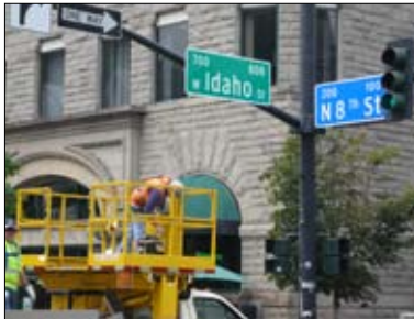
ACHD crews place new signs on 8th Street.
