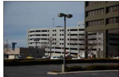
Boise Plaza's new garage in background.
