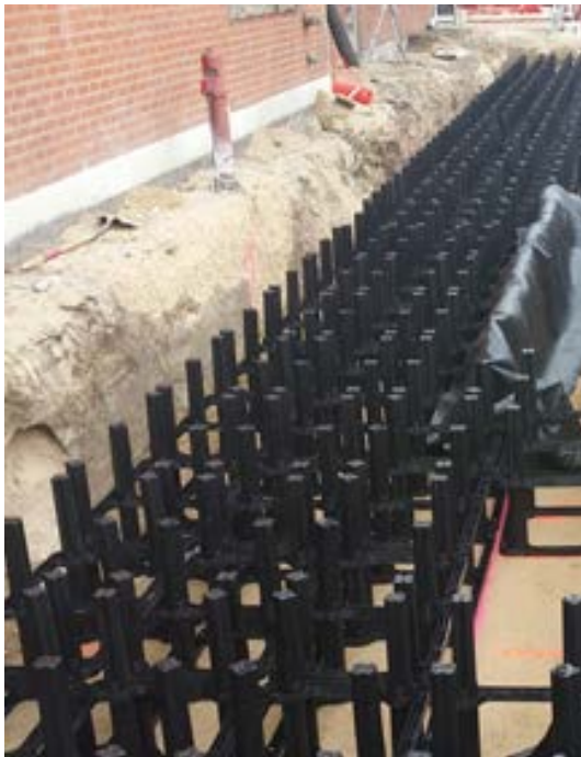
Suspended Paving Installation
